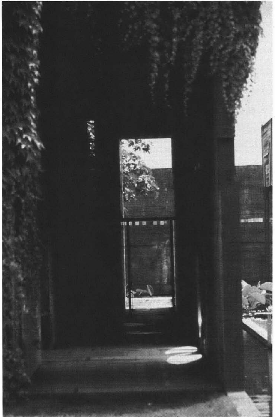
Figure 14. The bronze frame, but glass panels, of the door permits the visual extension of the cloister space out into the light of the pool. The mechanism of the door is concealed as much as possible on the inside of the tunnel, but the pulleys and counterweights become decorative elements on the exterior wall. Photograph by Richard Hansen.
